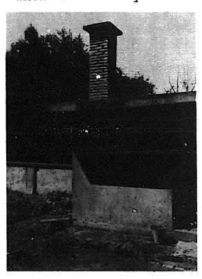
Good chimneys are made of masonry: bricks, stones or prefabricated chimney blocks with hollow spaces for insulation. Chimneys on flat roofs should be approx. 1.5 mtr above the roofing.
