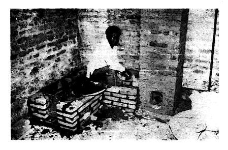
Construction of an improved cooking stove using bricks for the stove-walls and the chimney.
