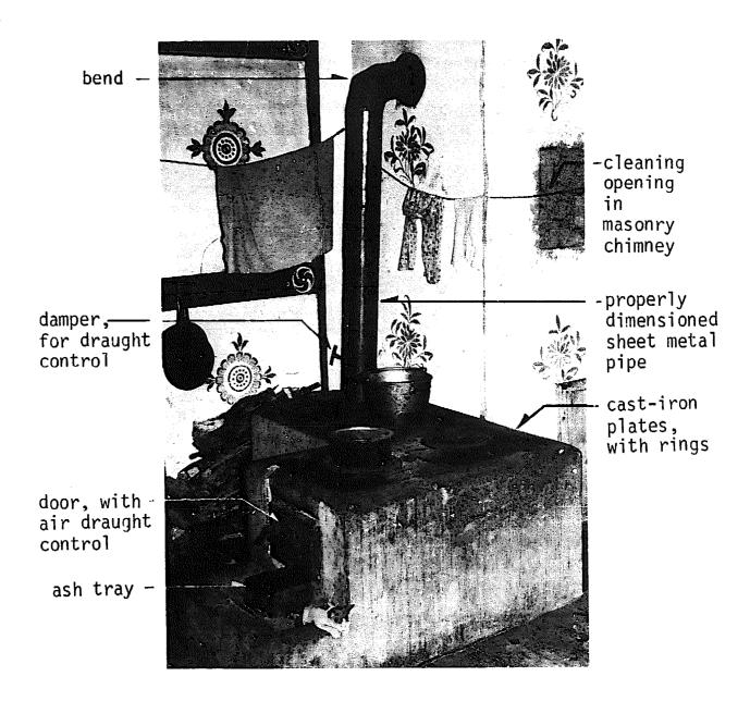
A "super cooking stove" in Bumthang, Bhutan. This stove, with its proper installation and incorporated cast-iron parts, provides fast and fuel-efficient cooking in a smoke-free kitchen.
