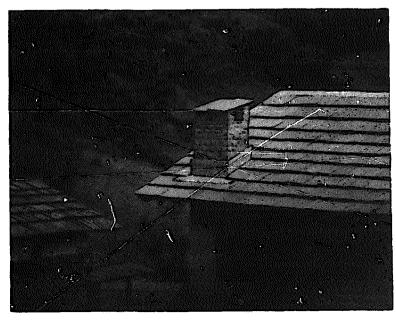
A chimney needs a proper flashing, to protect the house from leakages! This flashing is made of sheet metal by the Mechanical Training Center, Balaju, Kathmandu.
