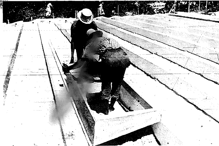
Fig 6: Finished curb and end walls with basin fill. The wooden frame is the guide used in levelling the basin fill in each of the twelve 6 foot long ponds that form one bay
