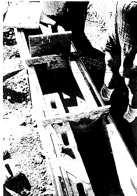
Fig 2: Special form used for positioning of concrete blocks and for moulding mortar and concrete into the shape of the gutters
