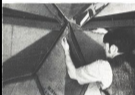
Flanged panels fasten together with stove bolts through drilled hardwood strips, as shown by Charles Krueger.
