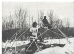
Conduit version of PS Sun Dome was so strong you could climb it, despite frost access gap. Weatherproof skin (and
