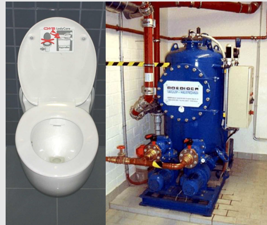
Figure 19: KfW office building “Ostarkade” (left); Vacuum toilet and pumping unit (right) (KfW)
