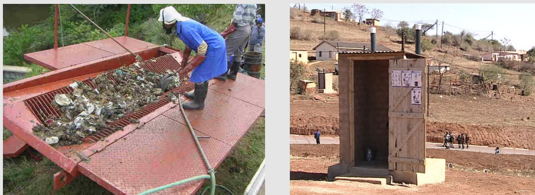
Figure 1: Emptying conventional pit toilets required special equipment (left picture) and turned out to be extremely costly - often exceeding 1000 Rand per pit. The urine diversion dehydration toilet (right picture) was selected by the communities as preferred solution after extensive awareness raising measures (Macleod 2005).
