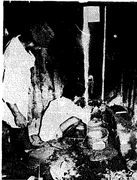
Trained installers at work in one of the rural kitchens.
