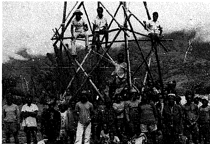
Fig. 2: Local Construction Crew
