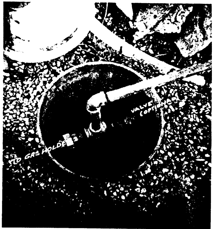
Figure 22A: Top view of trap. A valve is optional.
