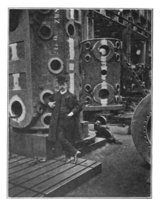
FIG. XII.-43. Cylinder casting, Nürnberg.
