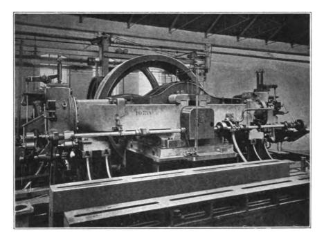
FIG. V.--7. Two-cylinder, ris-à-ris, single-acting, four-cycle Hornsby-Stockport Engine.
