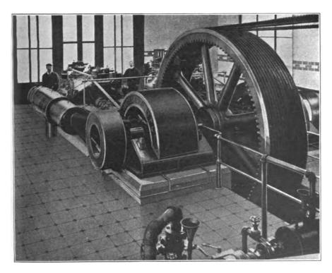
FIG. VIII.-9. 600 H.P. Mather & Platt Engine (Koerting type).
