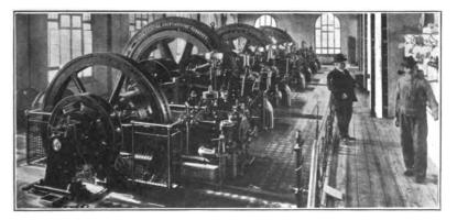
FIG. IV.—28. Six 300 H.P. Koerting four-cycle, single-acting, twin-engines at Julienhiitte Electricity Generating Station.
