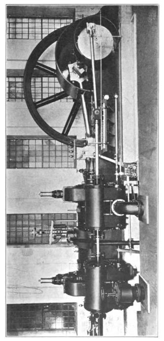
FIG. IV .- 25. Koerting two-cycle, double-acting Engine.
