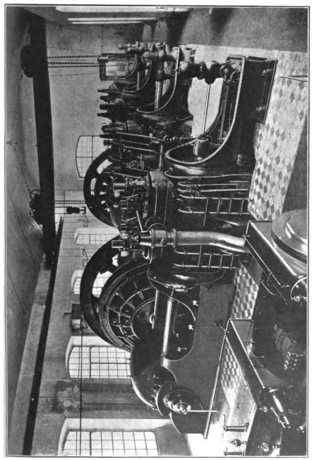
FIG. IV.--31. Two 1.100 H.P. twin-cylinder Nürnberg Engines and Dynamos at Micheville Steel Works.
