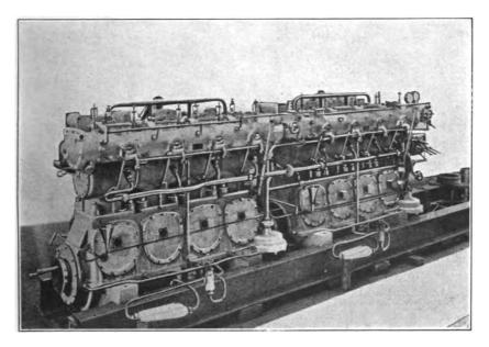
FIG. VII.-9. Thornycroft four-cycle, multi-cylinder Engine, for Submarine Vessels.
