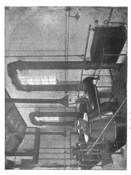
ing through the boiler; 71.3 per cent. was available for the engine, making the loss to the generator 24.4 per cent. Heat efficiency of the gas engine 19.3 per cent. per B.H.P.
