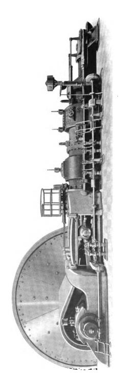
Fig. 90.—Borsig-Oechelhaueser Two-cycle Single Cylinder 1,800 H.P. Gas Engine.
