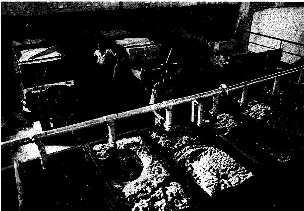
The factory's juice settling and filtration plant.
