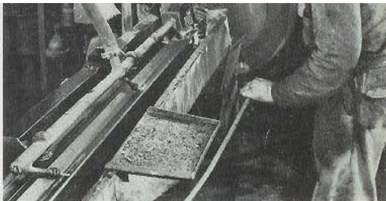
3. Extrusion of hollow carbons
